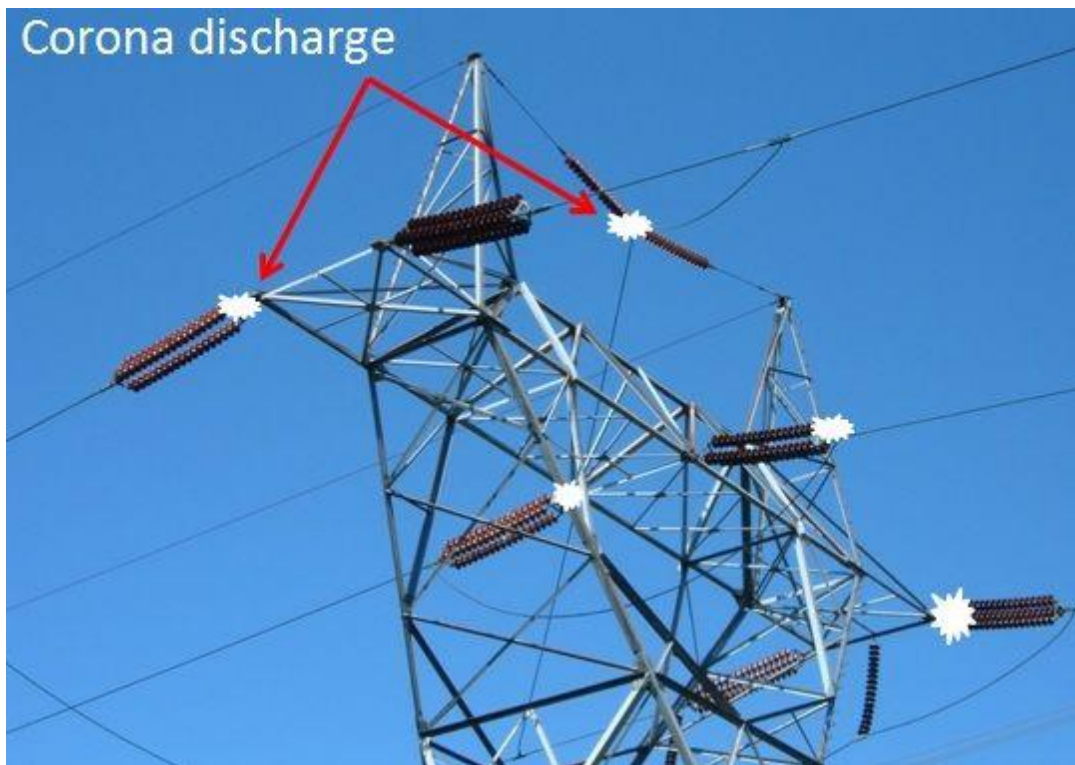
Corona effect mostly occurs at the sharp point of insulators.
