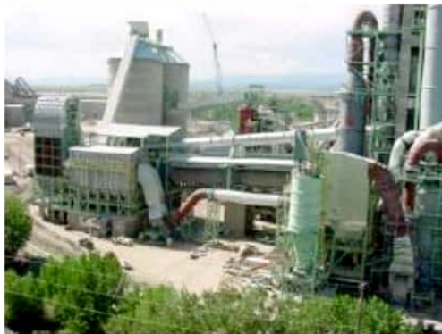
Kiln Line Overview
