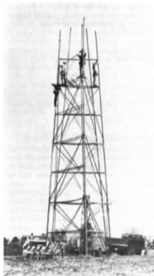
Bilby tower- construction
