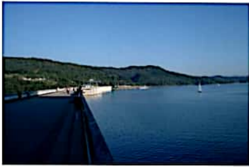
A power plant in Poland
